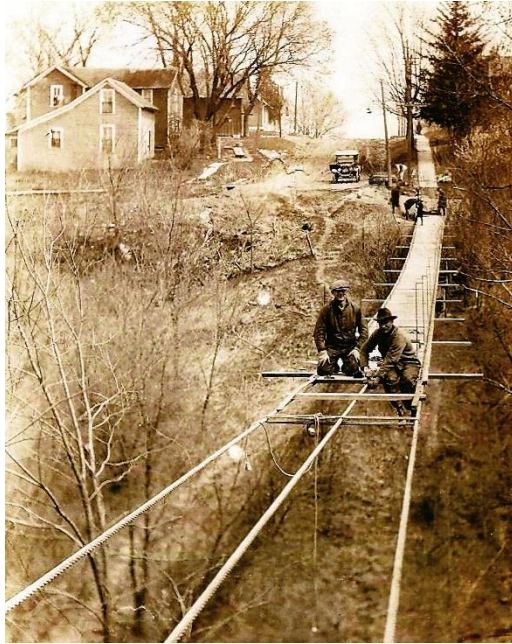
1922 Rebuilding of the bridge Harry Smith & R.C. Story
